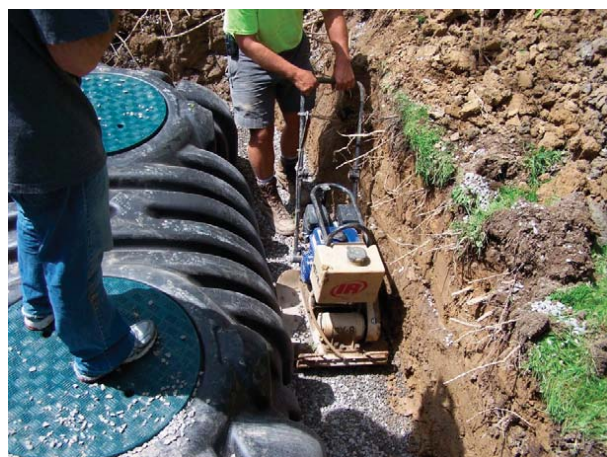
Photo 4.1.8-Example of mechanical compaction
