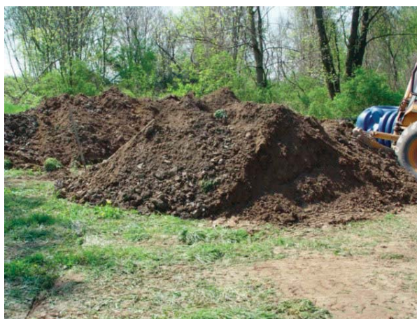
Photo 4.1.10-Example of backfilling material
