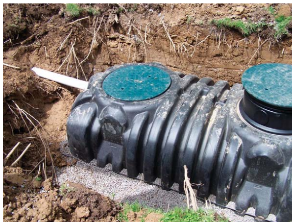
Photo 4.1.9-Uniform level distribution of material
