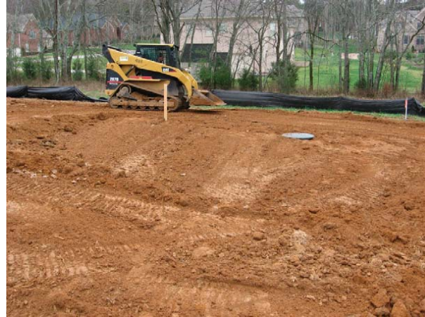
Photo 4.1.14-Example of final grading
